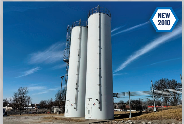
(2) 47.4" x 111" Diameter Silos (2010)
