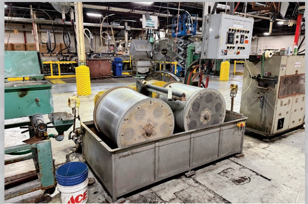
(7) IBT Two-Drum Coil / Accumulation Station
